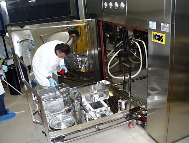
Washing unit entrance
